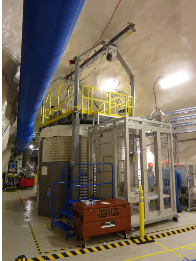
Figure 4.2: Photograph of the CUTE facility as seen from the ground level showing the close relation of the water tank and deck to the cleanroom where the cryostat can be moved to and from with the monorail crane mounted above.
