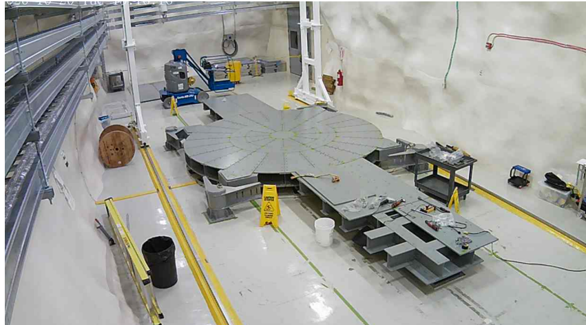
Figure 3.4: SuperCDMS Seismic Platform under construction in SNOLAB, 90% completed. Also seen in the photo are the gantry crane, and foundation for the cleanroom. Image source: [44]
